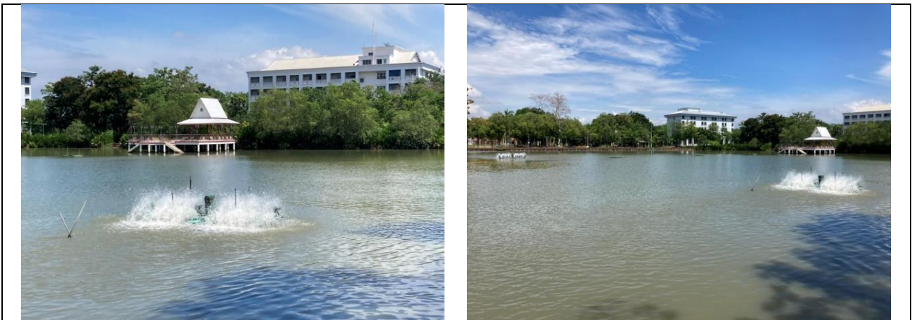
Aerated Lagoon and Paddle Wheel Aerator in NPRU
